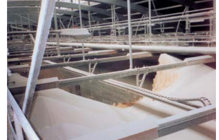
Bulk Material Crane
