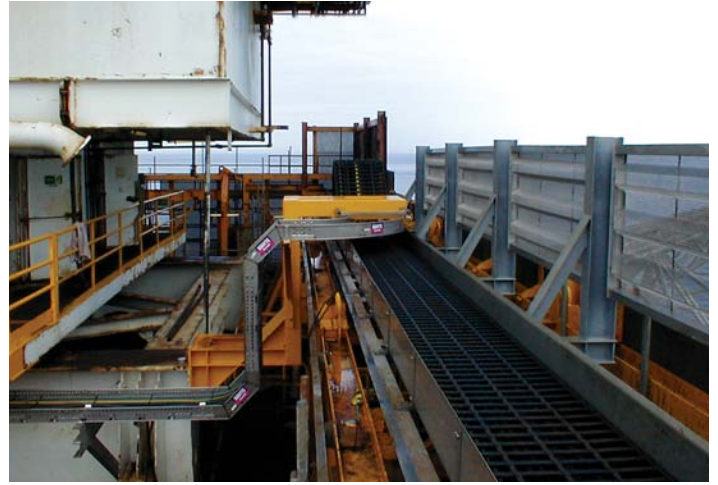
Rig skidding application in the Claymore, North Sea
